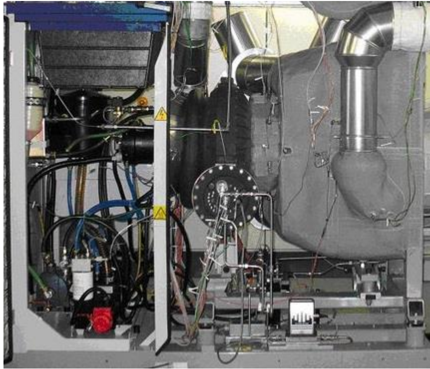
Turbec 100Kw micro turbine also fitted with exhaust heat recovery system
